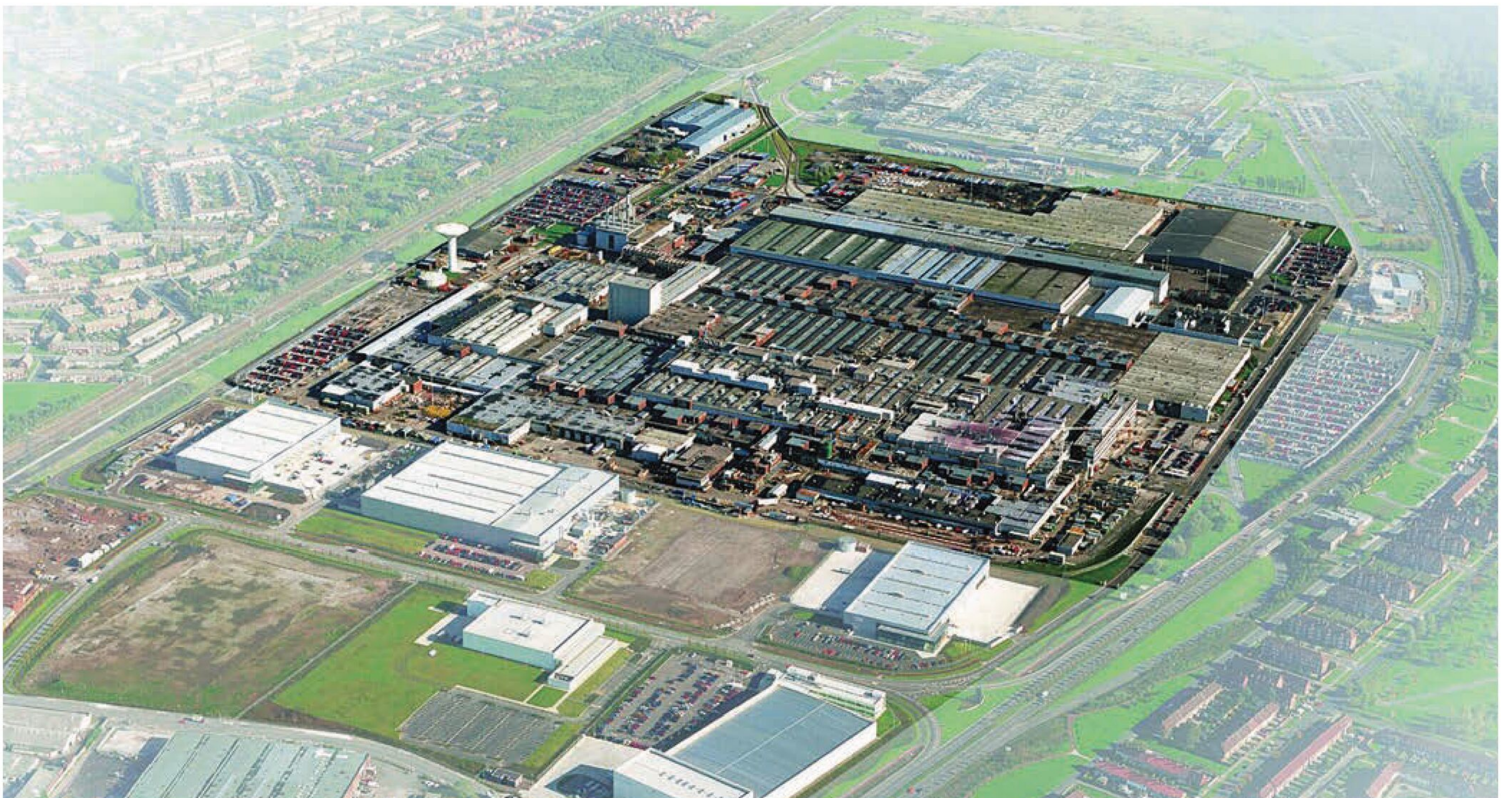
The plant at Halewood in 2006, during the days when it was building the X-Type.
